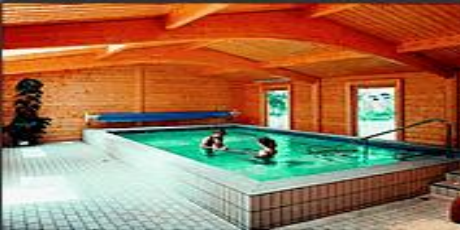
Pool room with glulam trusses and purlins Living area in oak
