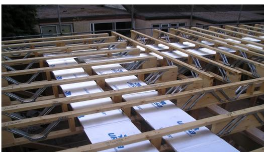
Using Ecojoist as the bottom chord increases the overall floor zone depth due to the requirement to rotate the top and bottom chords of the joist to match that of the remaining attic timbers. With the webs taken into account, the overall depth of the bottom chord increases from 222mm to 353mm.
